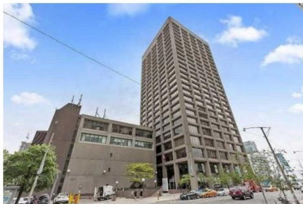
Pictured: The Building, which is made up of the Podium containing the three-story Warehouse (left) and the Office Tower (right).
